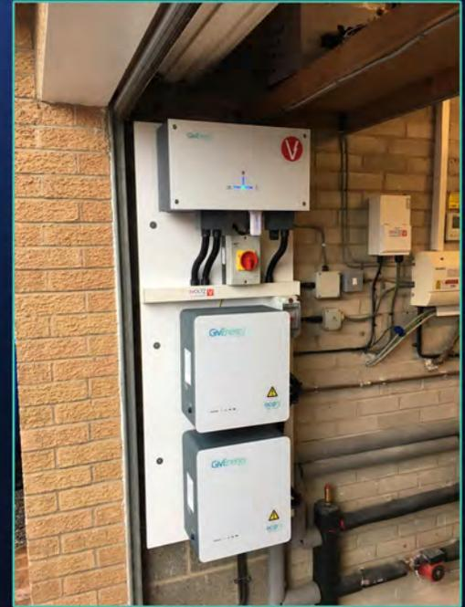
AC Coupled + 2x2.6kWh ECO Battery
